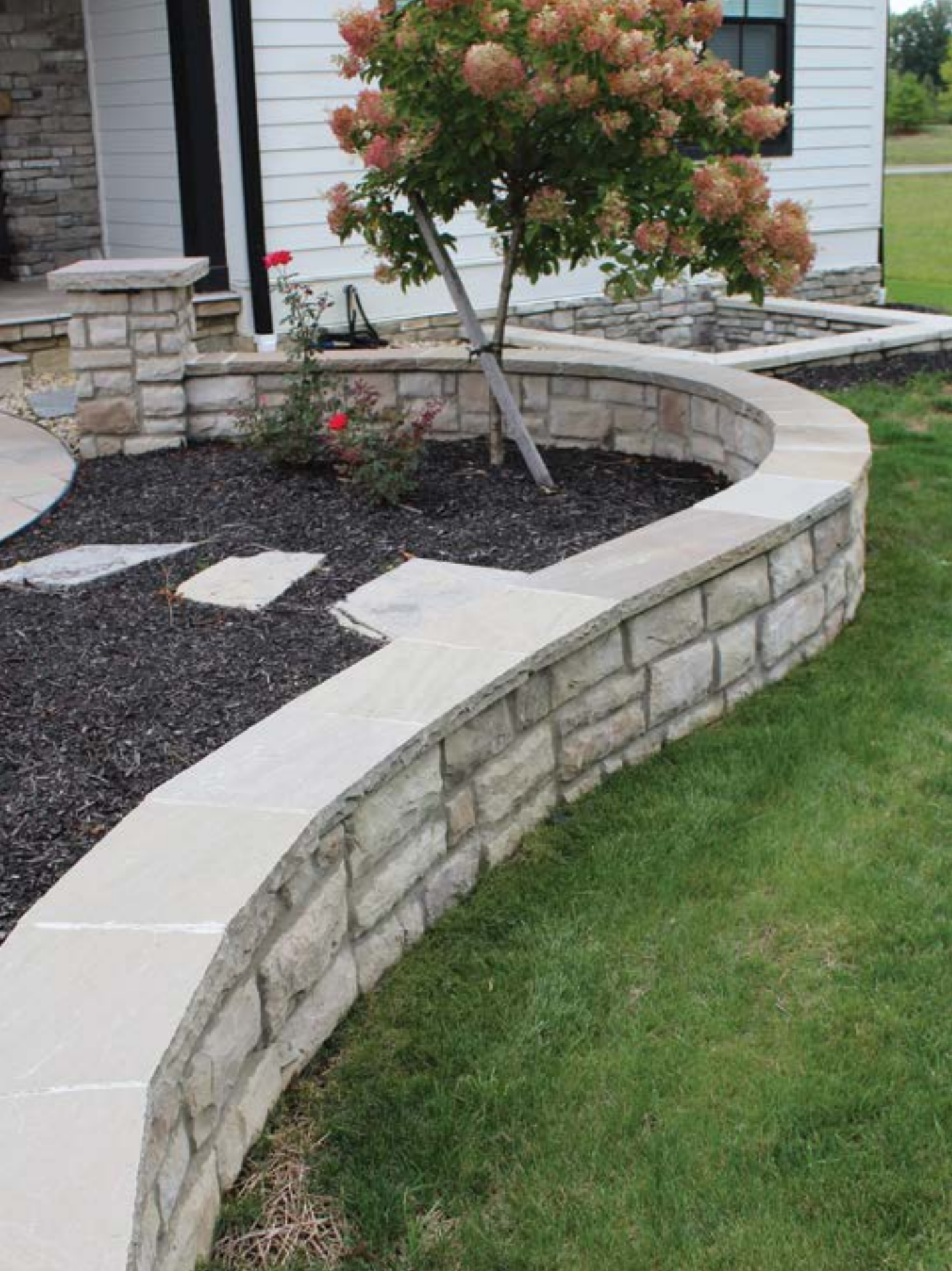
● Natural Stone Coping & Pier Cap
