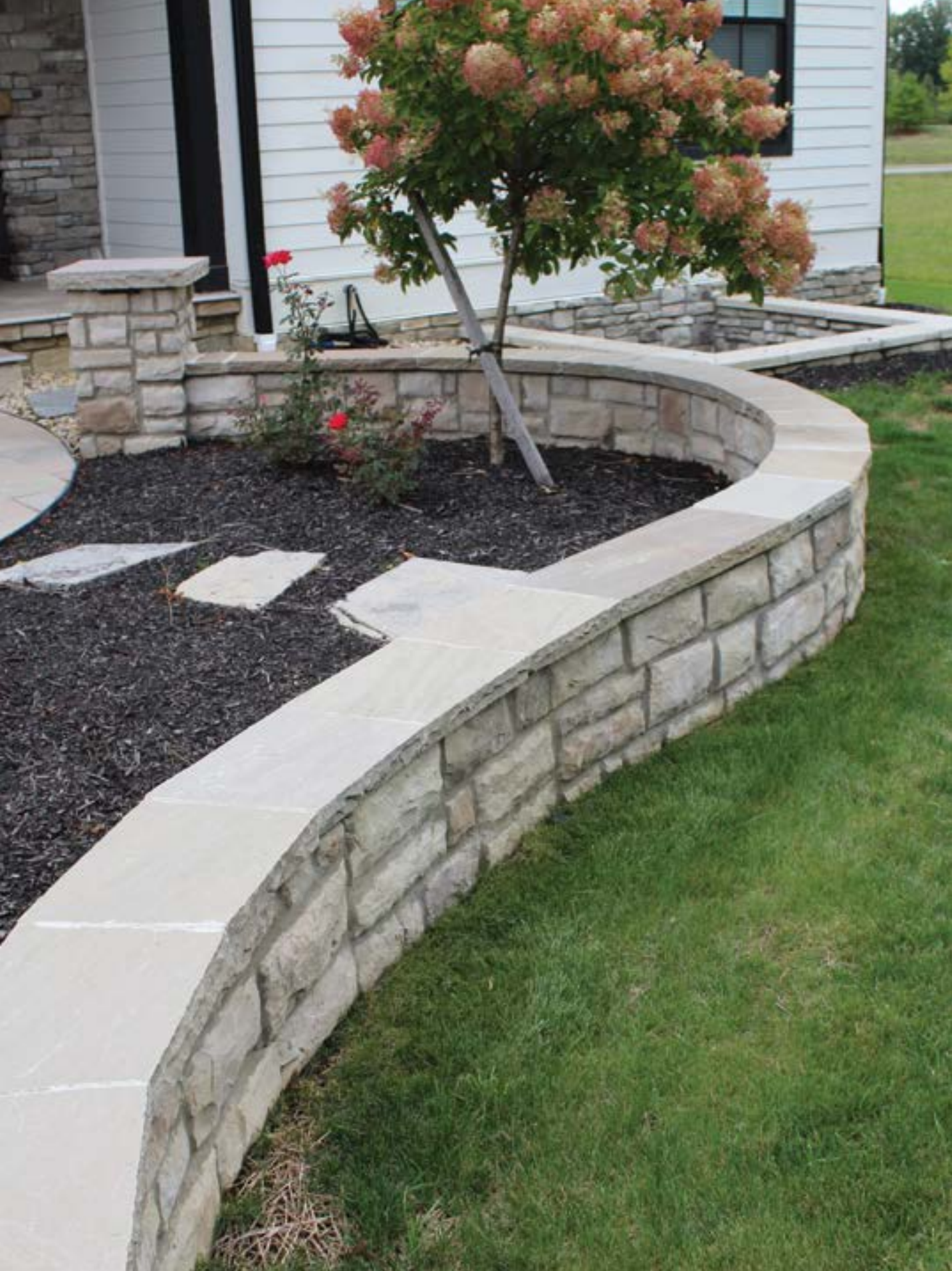
● Natural Stone Coping & Pier Cap
