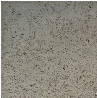
Light Sandblast Texture Natural Concrete Color
