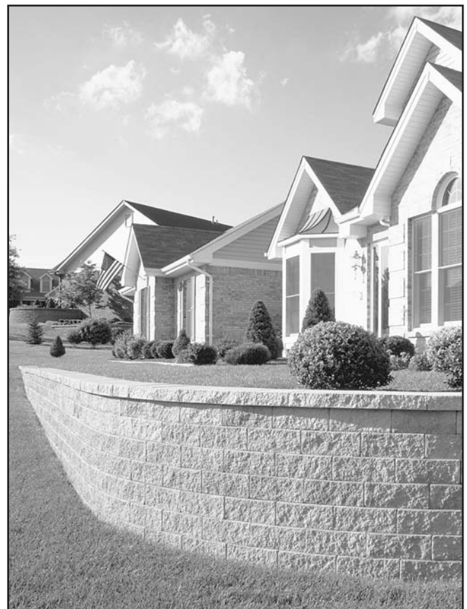
Careful base course planning for convex curves is important when building tight curves.
