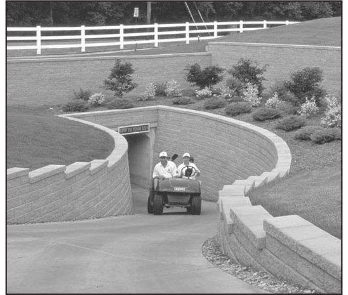
Build inside and outside curves with just one Standard VERSA-LOK unit—no specialty units needed.
