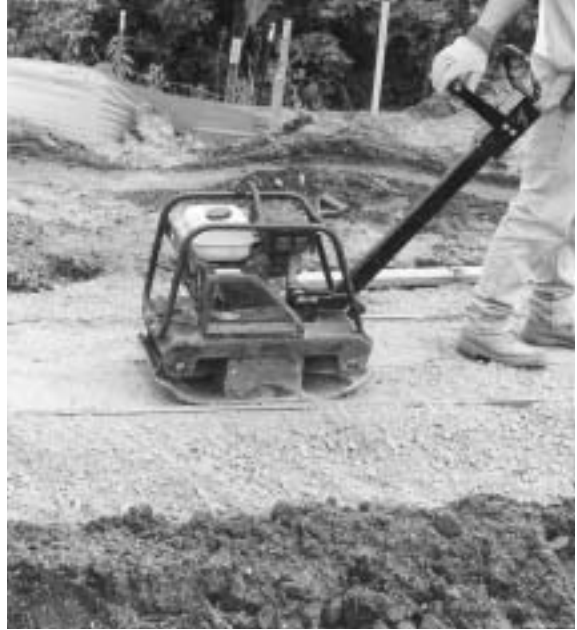
Compacted granular leveling pads provide stiff but flexible bases for Mosaic units.
