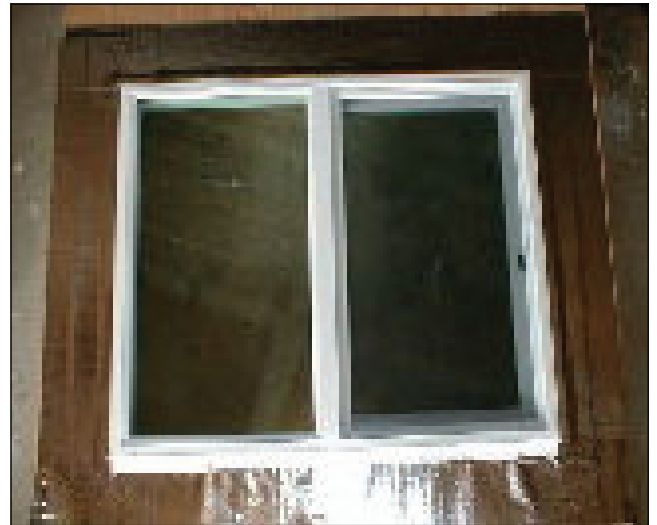
Install 6" flashing on sides.
