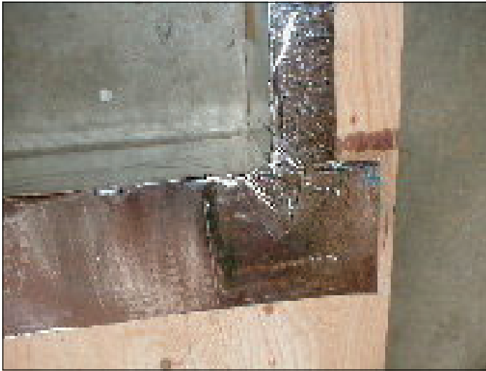
Install 12" flashing on bottom.
