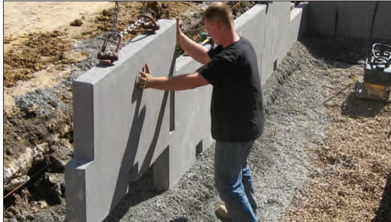
Step 3: Continue to install modules on first side.
