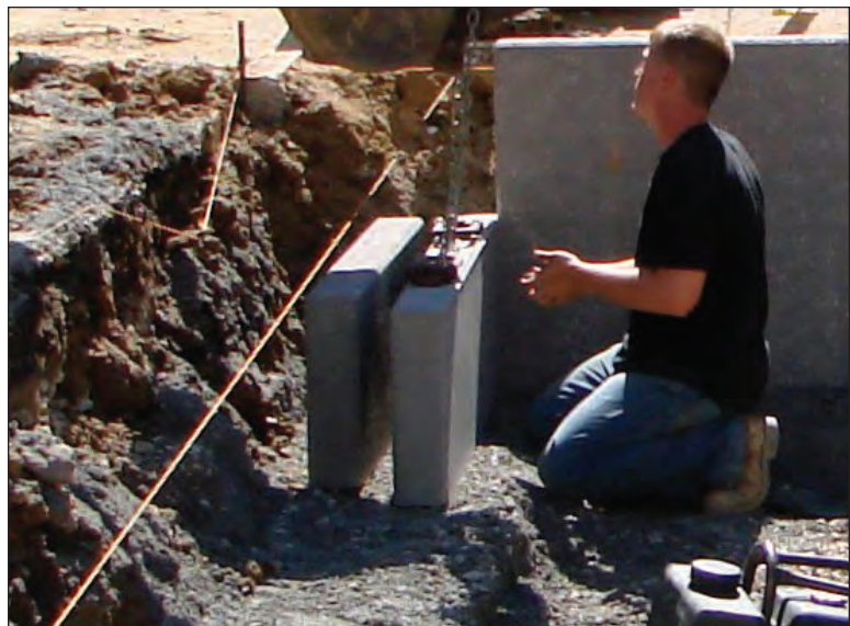
Step 2: Establish a corner by placing next module. Using a second T2 panel, install the foundation for the intake structure.
