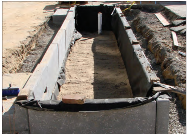
Step 9: Backfilling structure.
