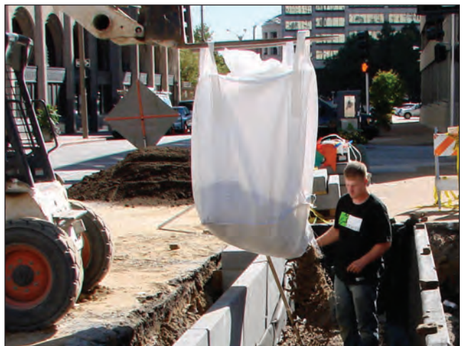
Step 10: Placing, Planting Soils.
