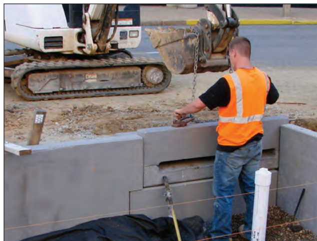
Step 7: Placement of second N•Module.
