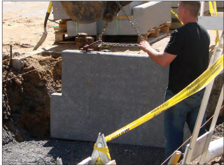
Step 1: Place and level first end Module
