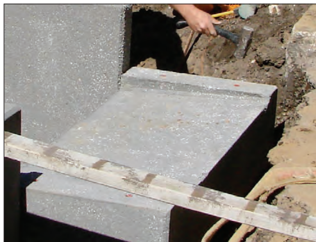
Step 8A: Placement of first N•Module.
