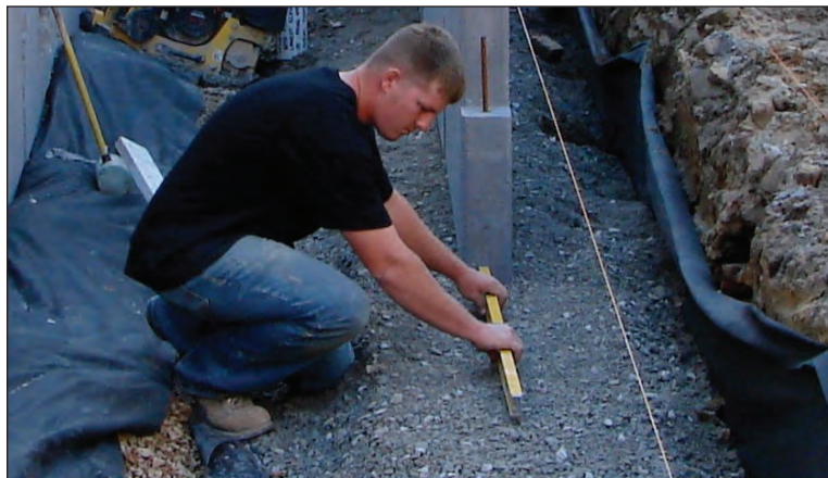
Step 5: Continue installing Modules on this side.
