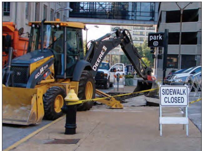
Site preparation and demolition
