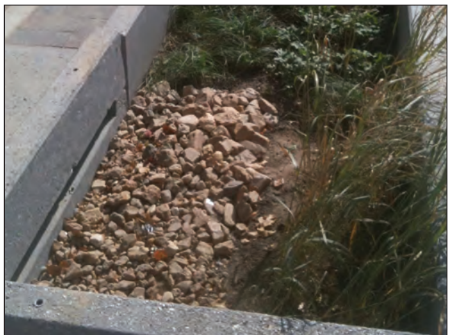
Erosion control at water intake
