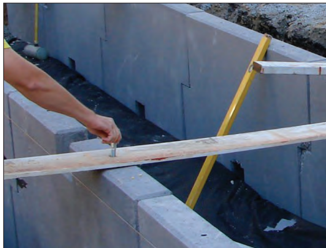
Installing temporary bracing
