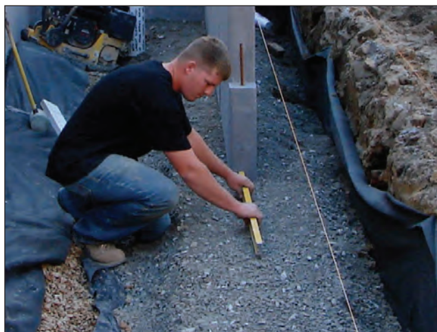
Confirming that base is level
