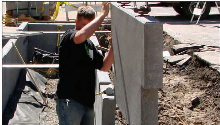
Step 7: Install the final side Module.
