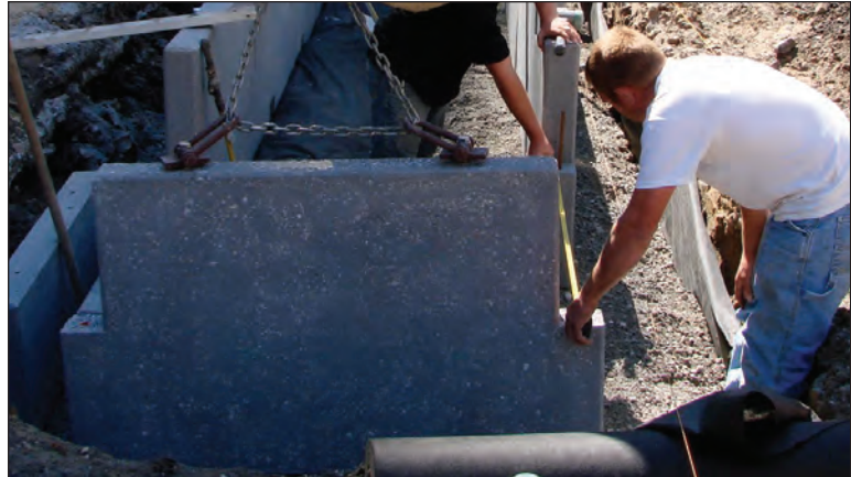
Step 6: Install the other end Module.
