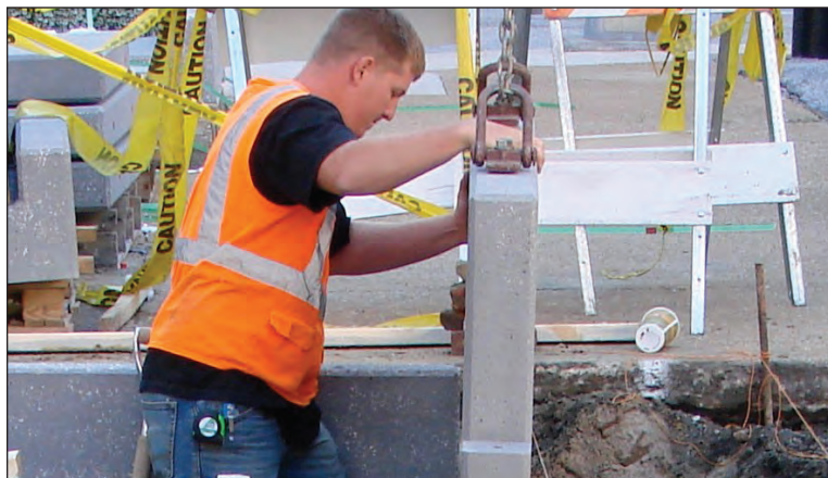
Step 4: Once the first side is completed, start installing the modules on the other side.
