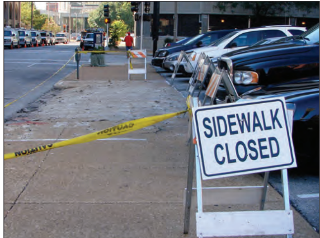
Place safety barriers
