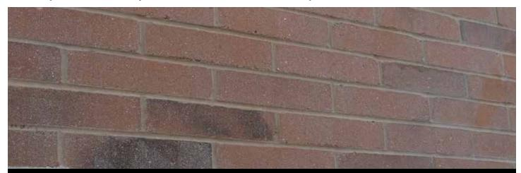
Cleaned Wall Section showing discoloration and damage due to use of high pressure rinse - note the wand marks where the wall was particularly hard hit (water pressure was 500 psi)
