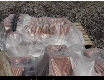
Materials should be stored on pallets and protected from the elements while stored on site
