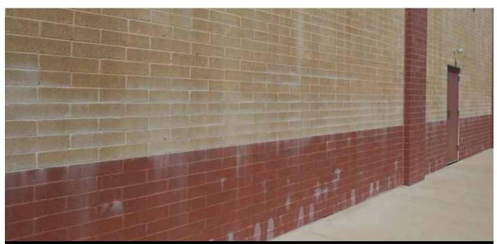
A failure to protect the exposed wall tops from rain during construction can lead to the wall's empty cores filling with water, which as it drains out of the wall leaches salts from the concrete which results in efflorescence forming on the exterior. This makes cleaning the wall much more difficult
