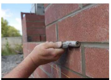
Tool Joints when they have reached thumb-print hardness for best results
