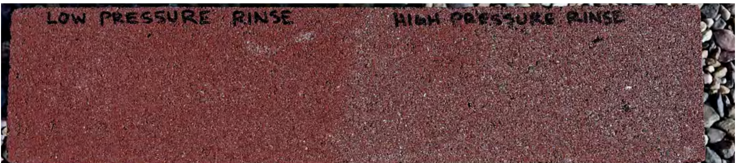
This Masonry Unit was cleaned with EaCo Chem NMD-80 using standard application methods, but the left side was rinsed using low water pressure and the right side was rinsed with high water pressure
