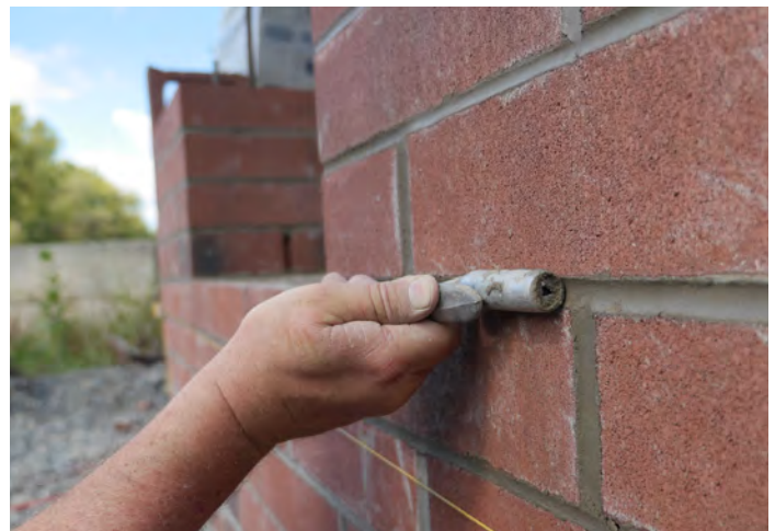
Tool Joints when they have reached thumb-print hardness for best results
