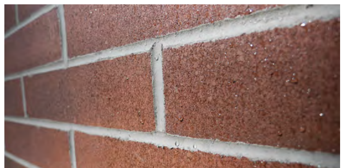
Integral Water Repellent and Post-Applied Sealant Provide Excellent Weather Protection
