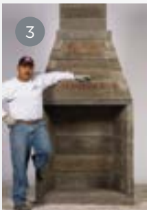
3 Install firebrick and fireplace is complete.
