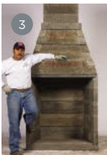
3 Install firebrick and fireplace is complete.
