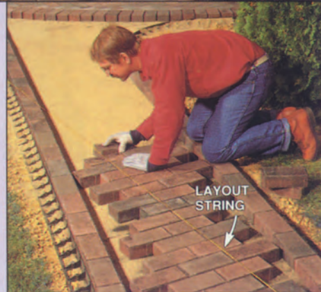
ANGLE CUT EVERY OTHER BORDER PAVER AT CURVE
