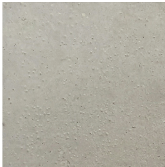
Smooth As-Cast Surface Natural Concrete Color
