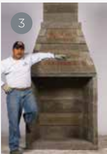
3 Install firebrick and fireplace is complete.
