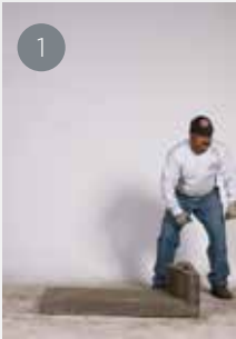
1 Set base plate on non-combustible foundation.
