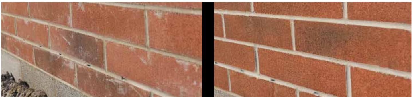
This Wall Was Cleaned within 7 Days of Construction Using Low Pressure Application and Rinsing
