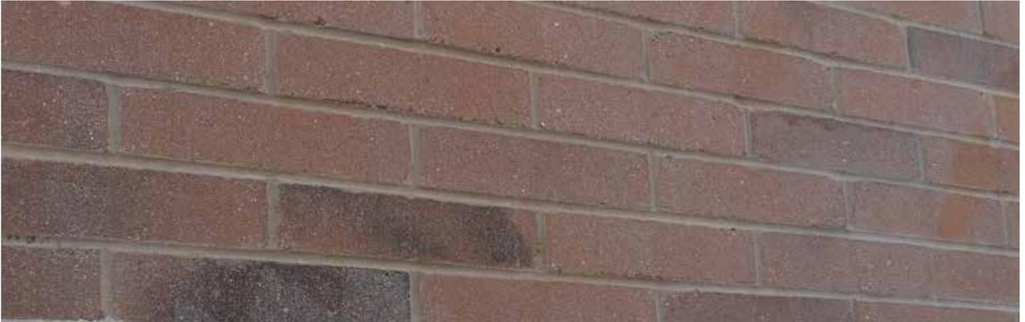
Cleaned Wall Section showing discoloration and damage due to use of high pressure rinse - note the wand marks where the wall was particularly hard hit (water pressure was 500 psi)
