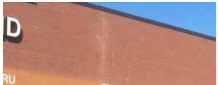
Staining from Saw Dust Left on Block
