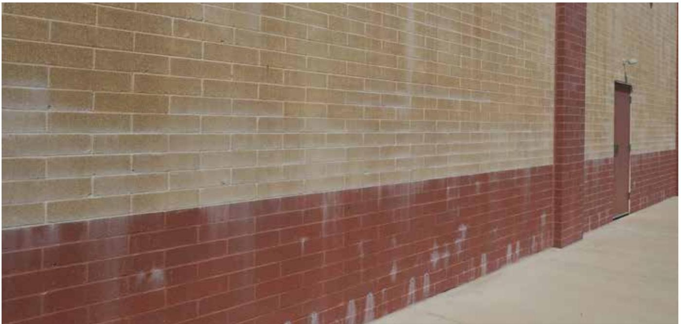
A failure to protect the exposed wall tops from rain during construction can lead to the wall's empty cores filling with water, which as it drains out of the wall leaches salts from the concrete which results in efflorescence forming on the exterior. This makes cleaning the wall much more difficult
