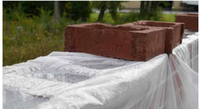
Wall top tarped to protect against rain during a break in construction.
